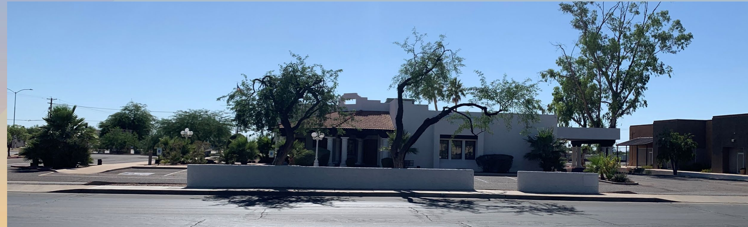
Looking west from 57 th Street
