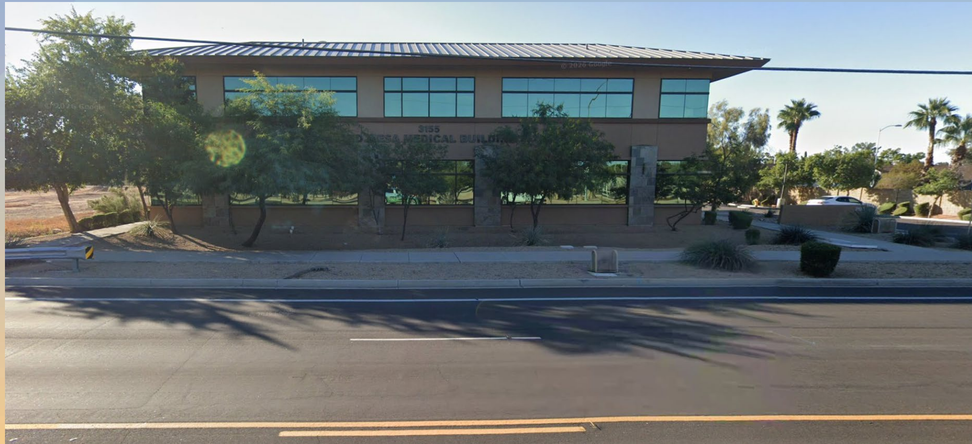
Looking south towards the project site
