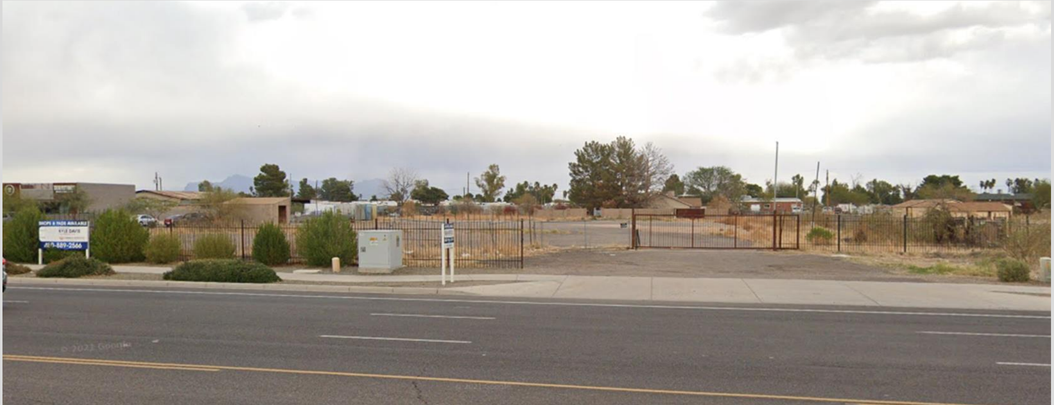
Looking east from Power Road
