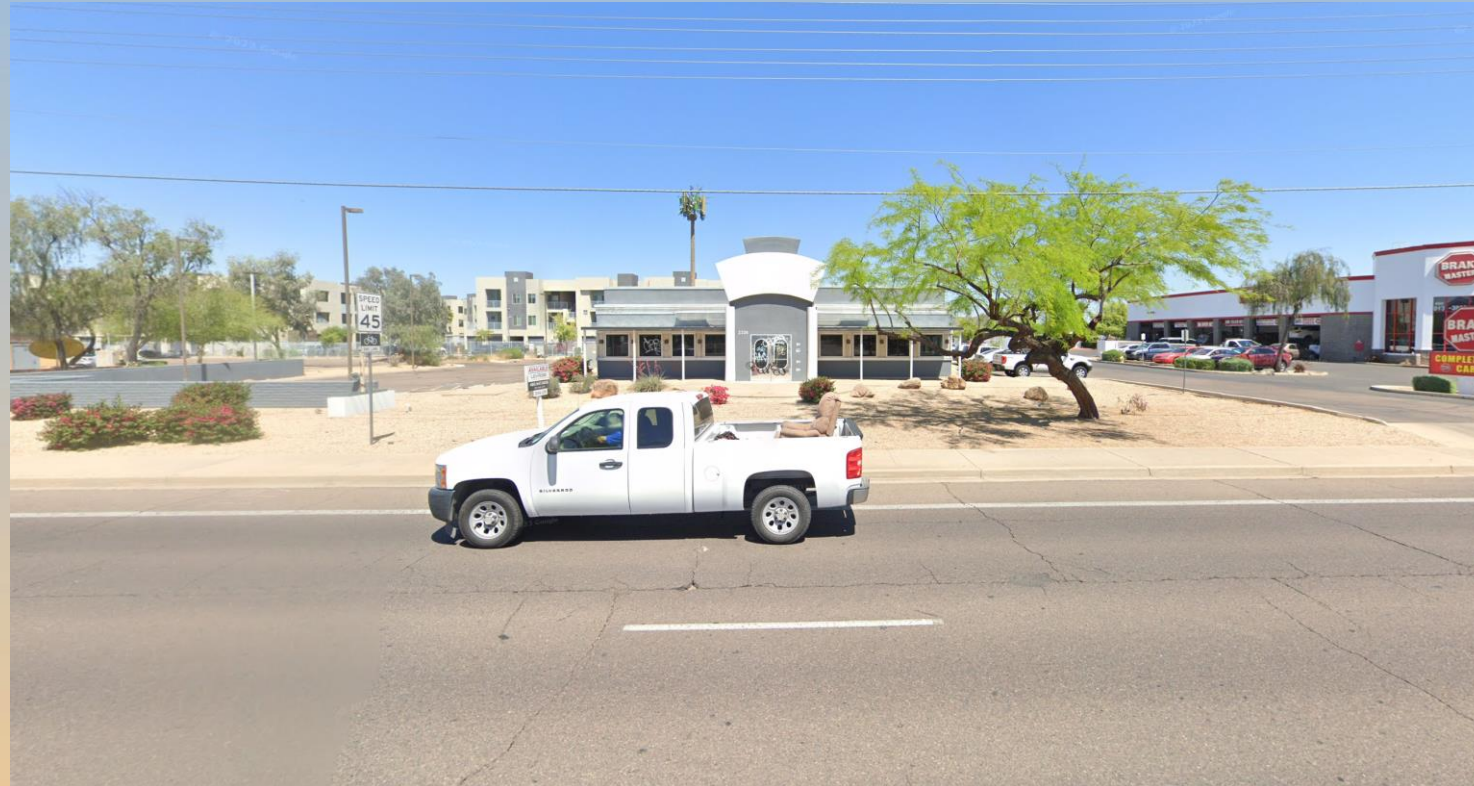
Looking north at the site from Baseline Road
