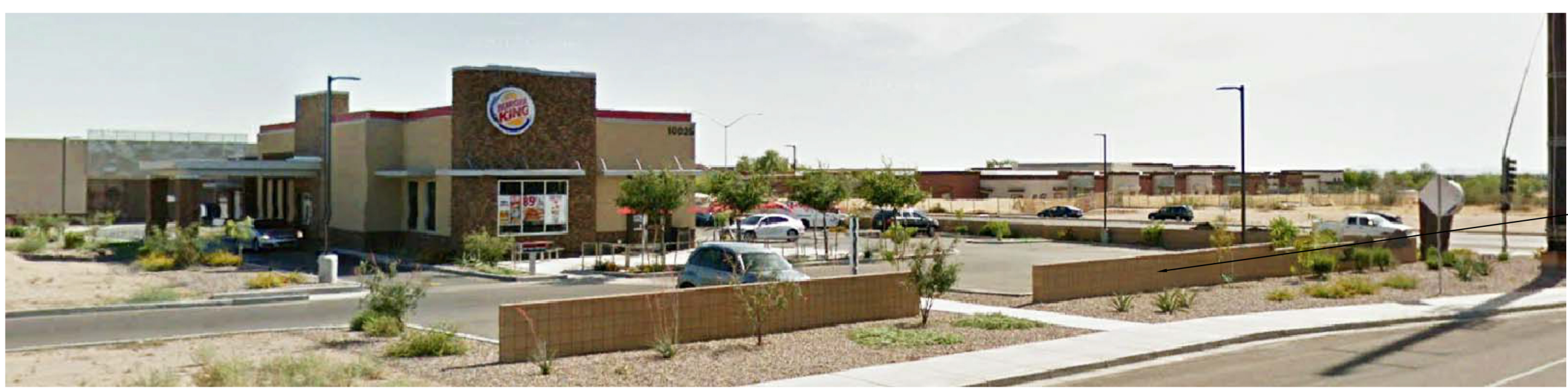
EXISTING SITE PHOTO VIEWING THE EXISTING PARKING SCREEN WALL ALONG SOUTHERN AVE. AT BURGER KING PROPERTY.
