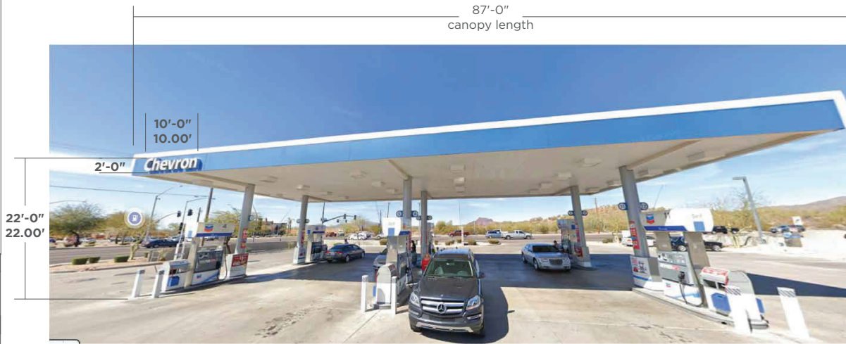
Existing South Elevation View
