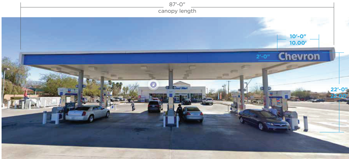
Existing North Elevation View
