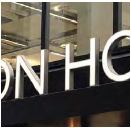
Channel Letter Mounted on Canopy Face with Hidden Raceway
