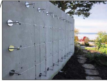
STAR JASMINE TO BE SHOWN ON STAINLESS CABLE TRELLIS AS SHOWN IN PHASE TO THE LEFT SCS CABLE SOLUTIONS, LLC 800-380-4198 WWW.STAINLESSCABLESOLUTIONS.COM
