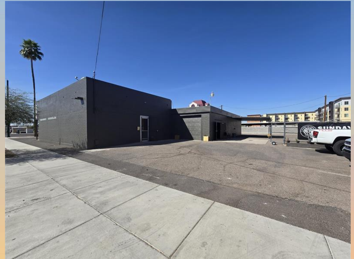
South and East Side
