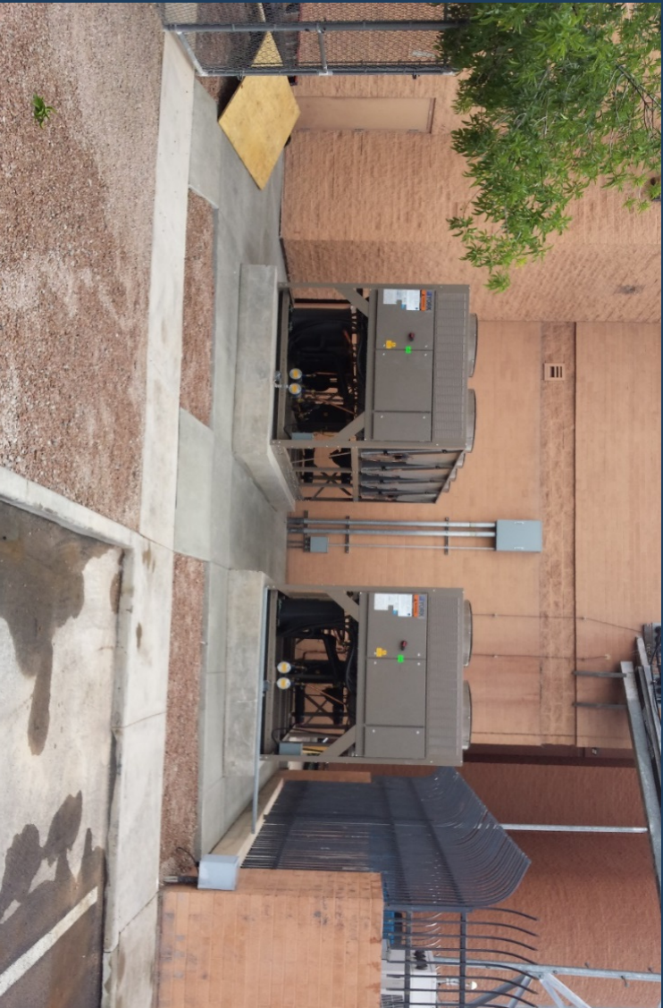
Required HVAC (Exist. Communications Bldg. Chillers)
