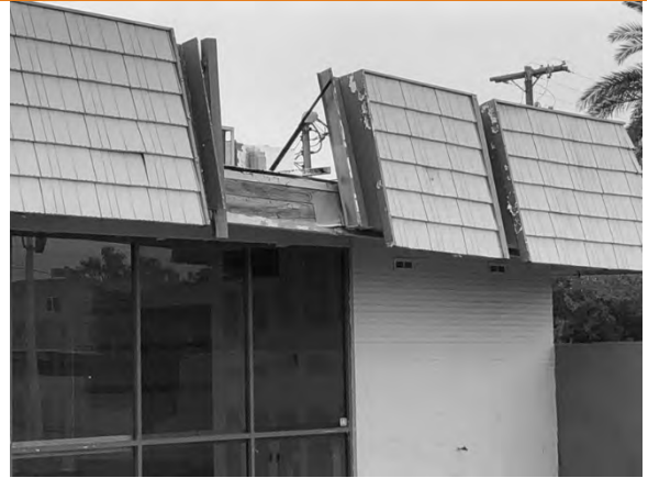
Portion of roof collapsed and in need of replacement.
