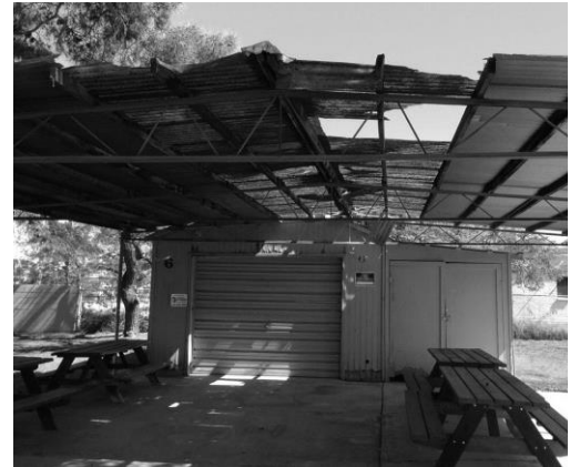
Example of a severely damaged, partially collapsed, unstable roof.
