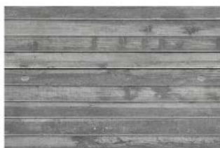
BOARD FORMED CONCRETE GRAY CONCRETE WITH 2x6 ROUGH SAWN WOOD FRAME TO ACHIEVE LOOK
