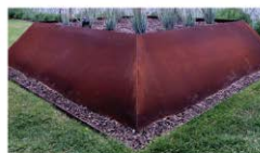
ANGLED CORTEN STEEL NATURAL FINISH, TO RUST WITH AGE
