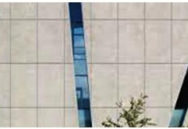
Concrete Tilt Panels
