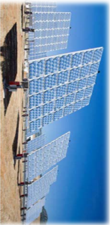
Brown Rd - 70 KW SolFocus Concentrated Photo Voltaic (CPV) Dual Tracking System. City owned!
