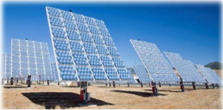
Brown Rd - 70 KW SolFocus Concentrated Photo Voltaic (CPV) Dual Tracking System. City owned!
