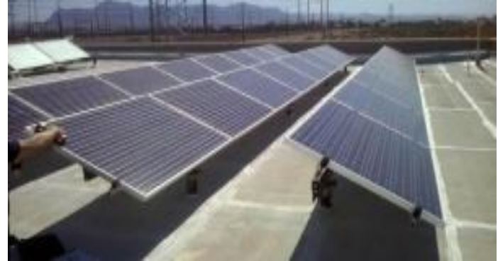
FS 219 - 5 KW Photo Voltaic Roof Mount System and Solar Hot Water
