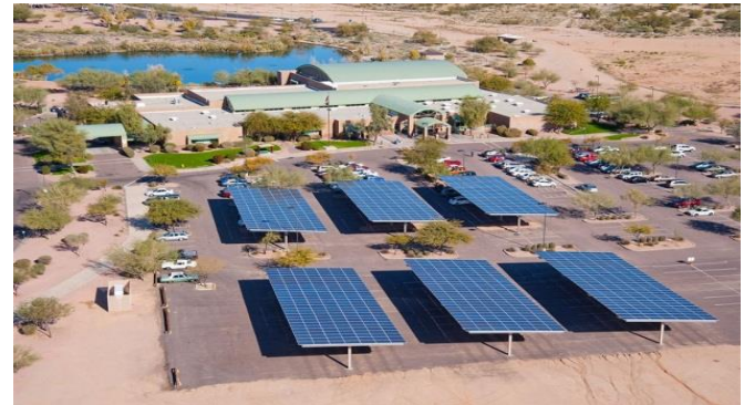
Multi Gen Center - 294 KW Photo Voltaic Carport Mount System
