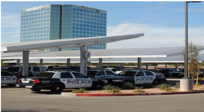
Fiesta PD - 272 KW Photo Voltaic Carport Mount System
