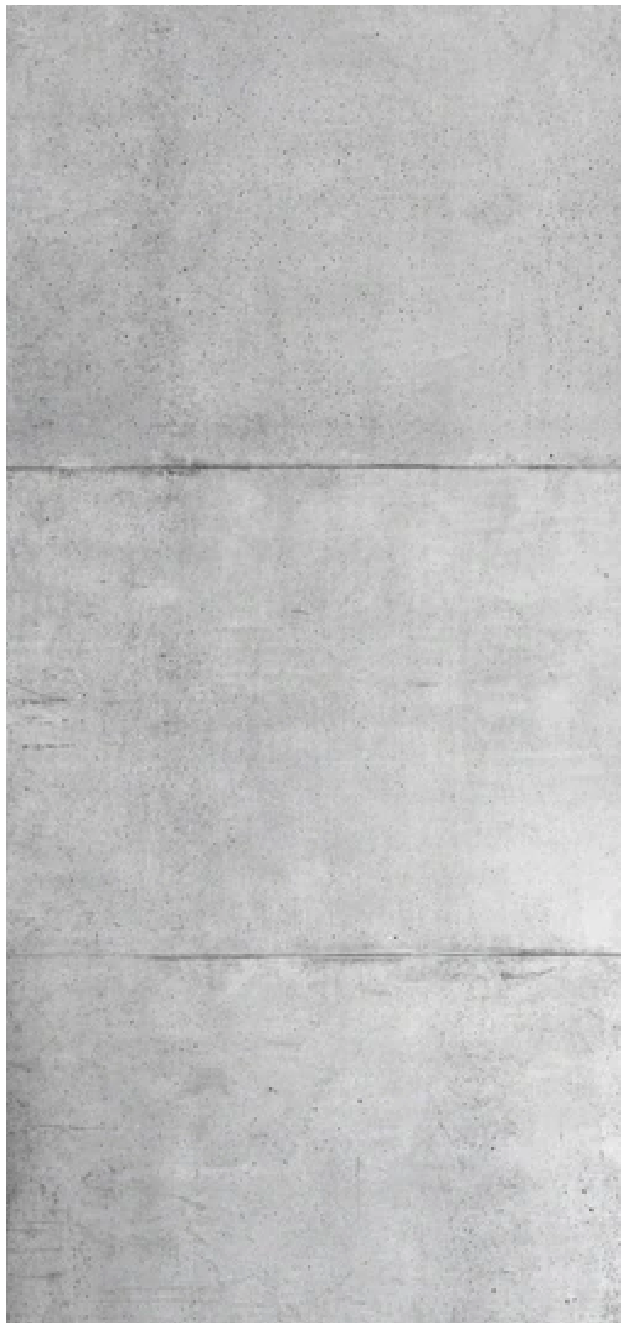
Exposed Concrete : Columns
